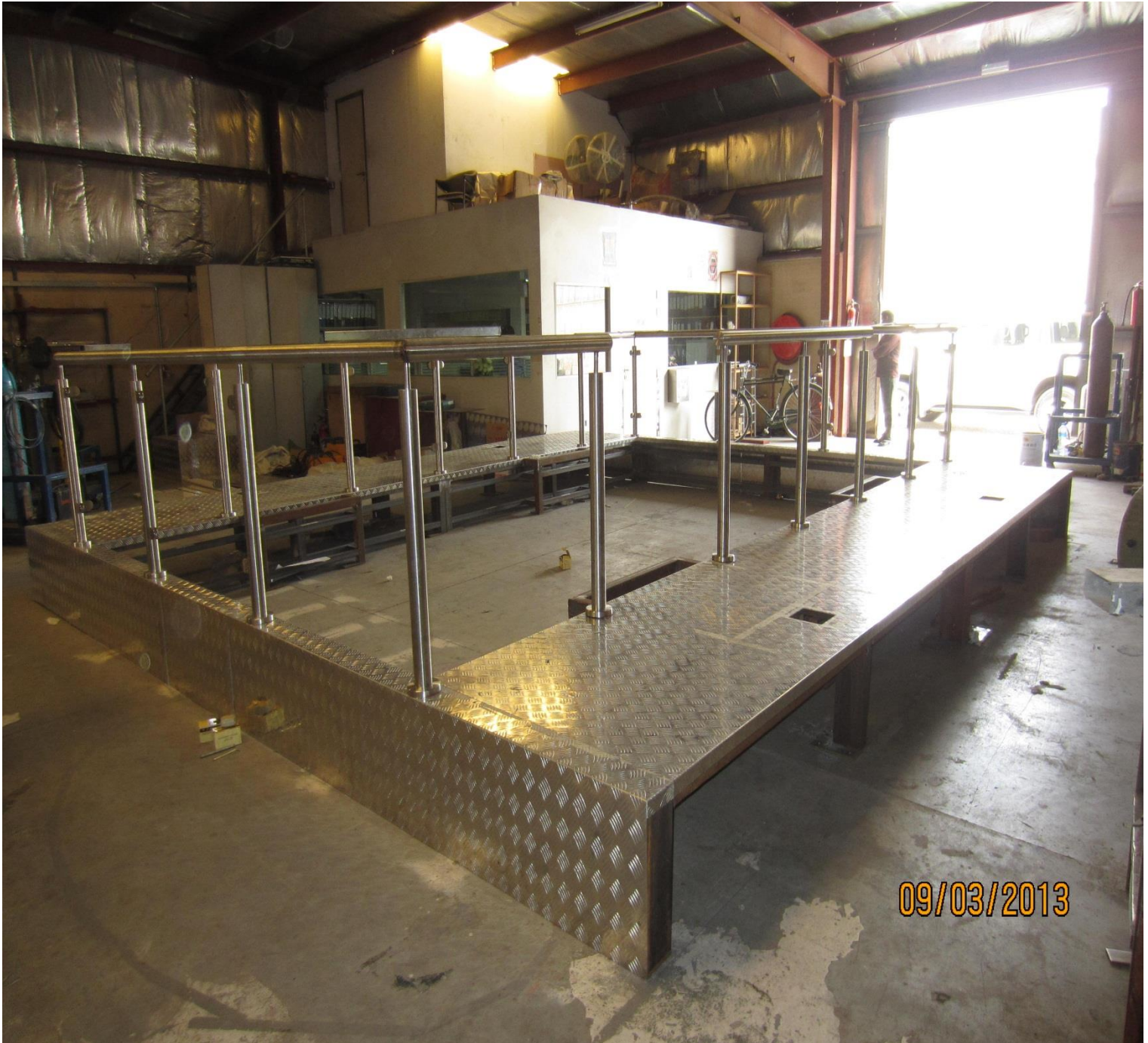
Steel Floor- City walk - Dubai
