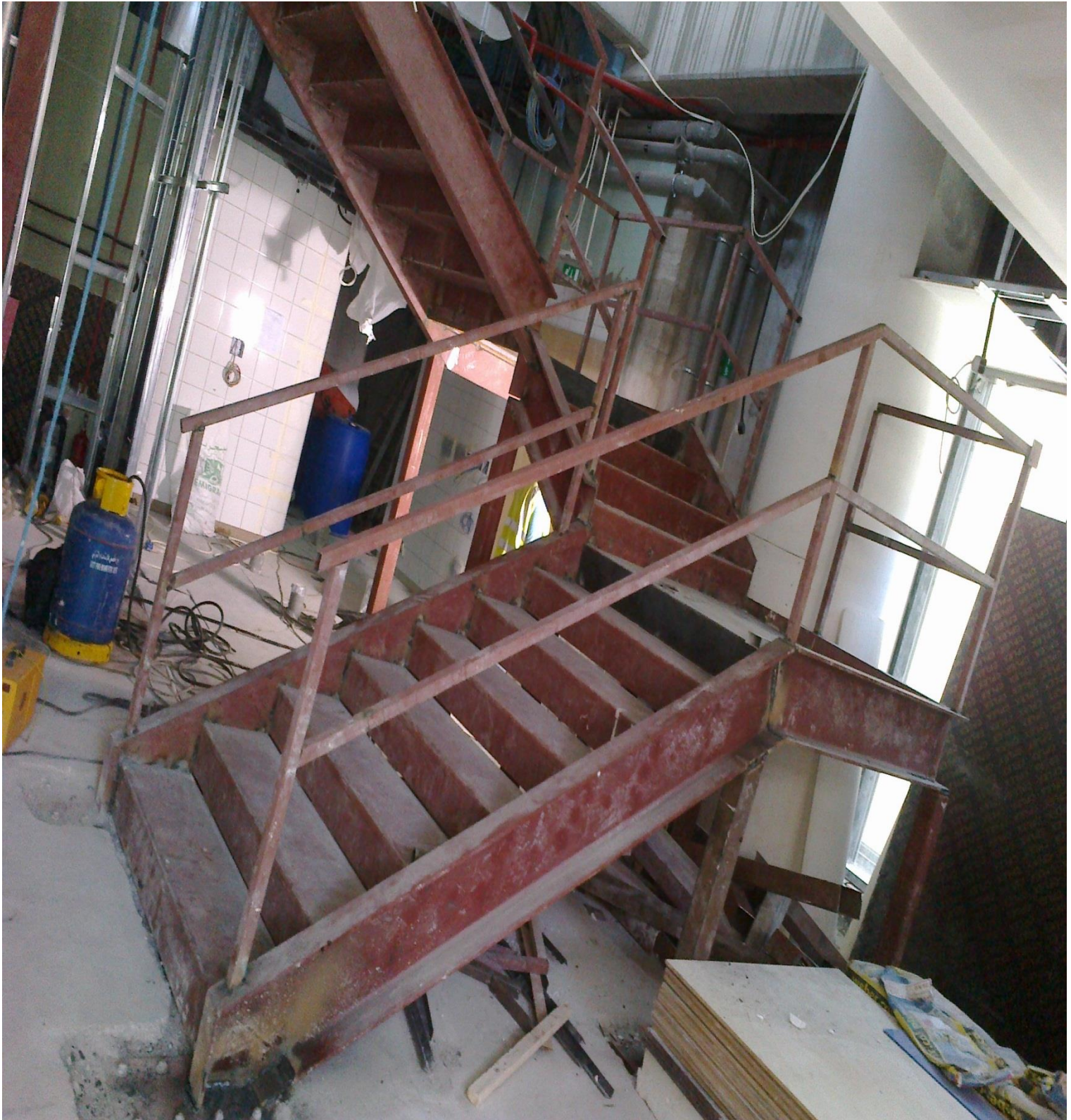
Steel Stair- Villa at Emirates Hill- Dubai
