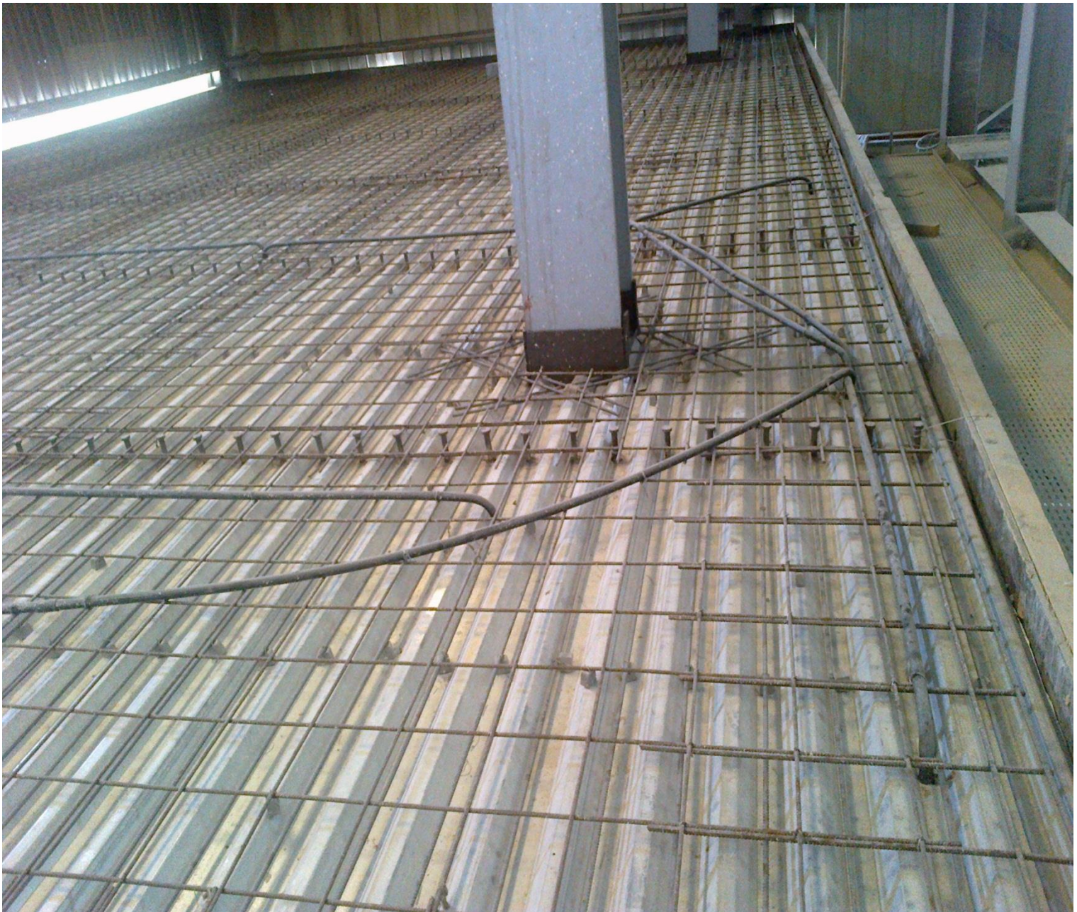
Mezzanine floor - Coast Flour Mill- Jebel Ali Free zone
