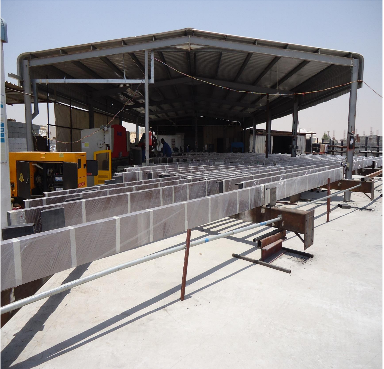
Steel Structure- New York University- Abu Dhabi
