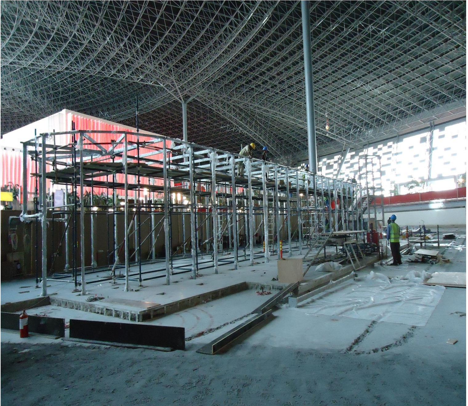
Steel structure- Ferrari Abu Dhabi
