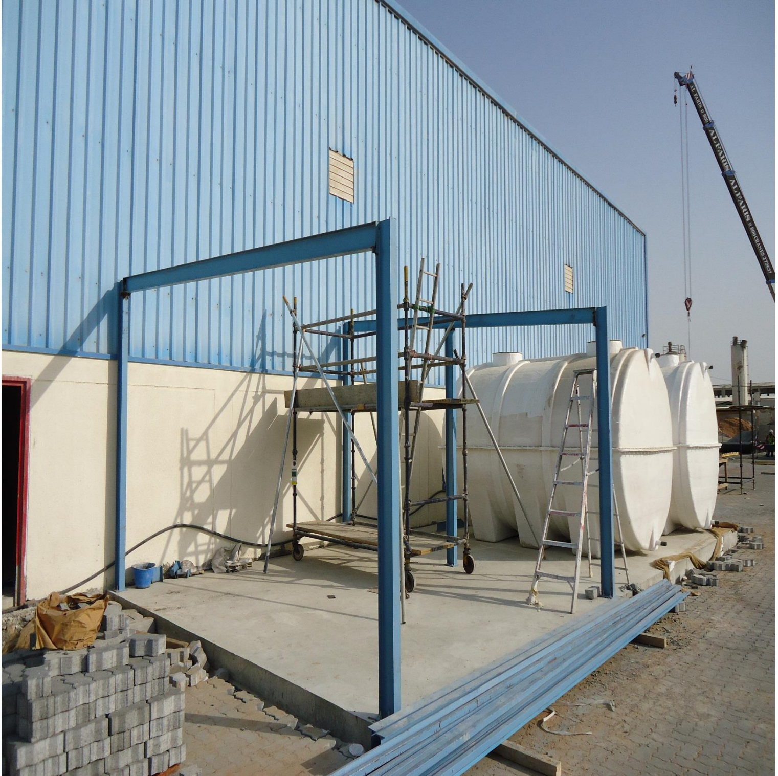
Steel Structure- Keys Factory- Techno Park- Dubai
