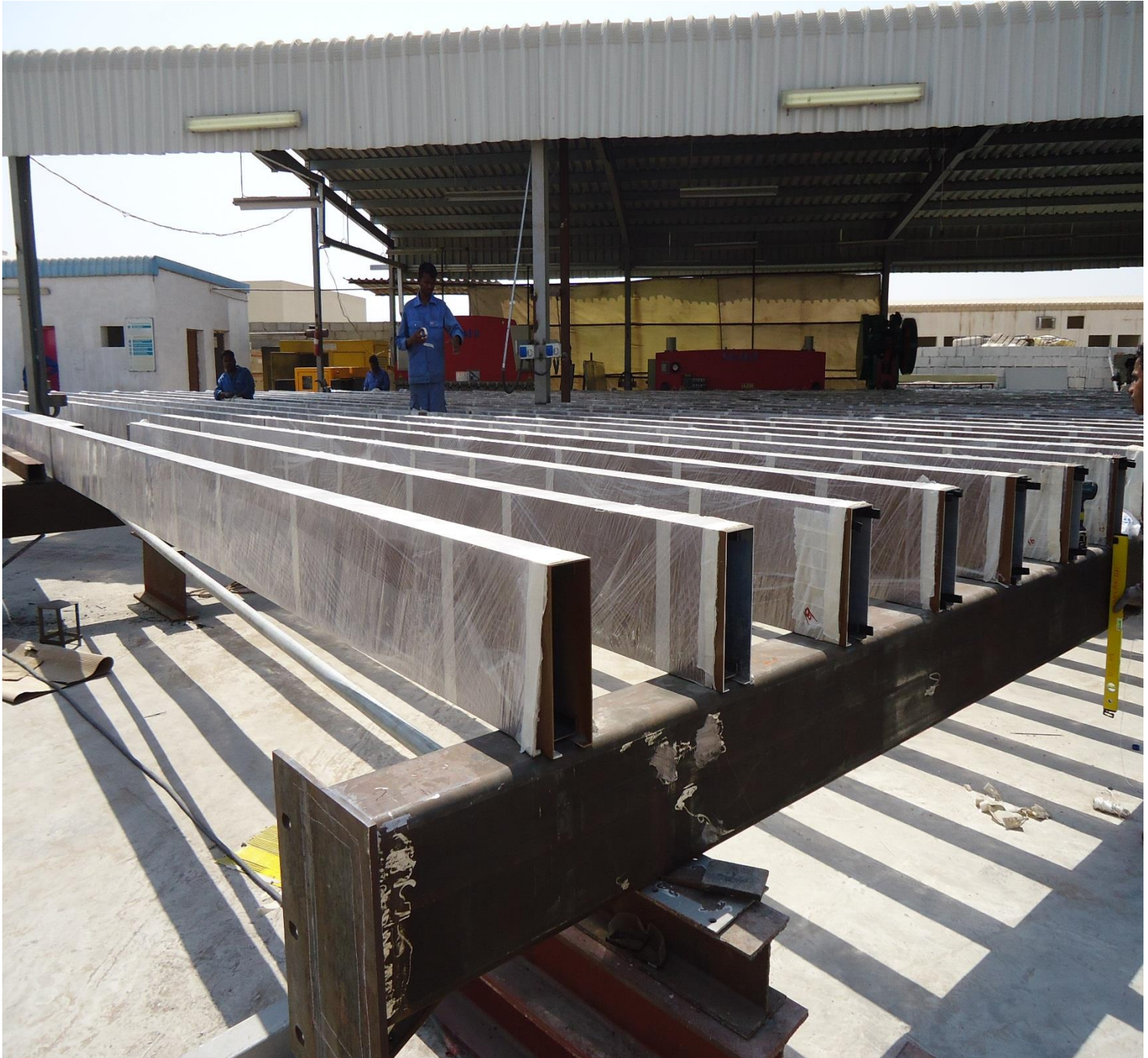
Steel Structure- New York University- Abu Dhabi (2)
